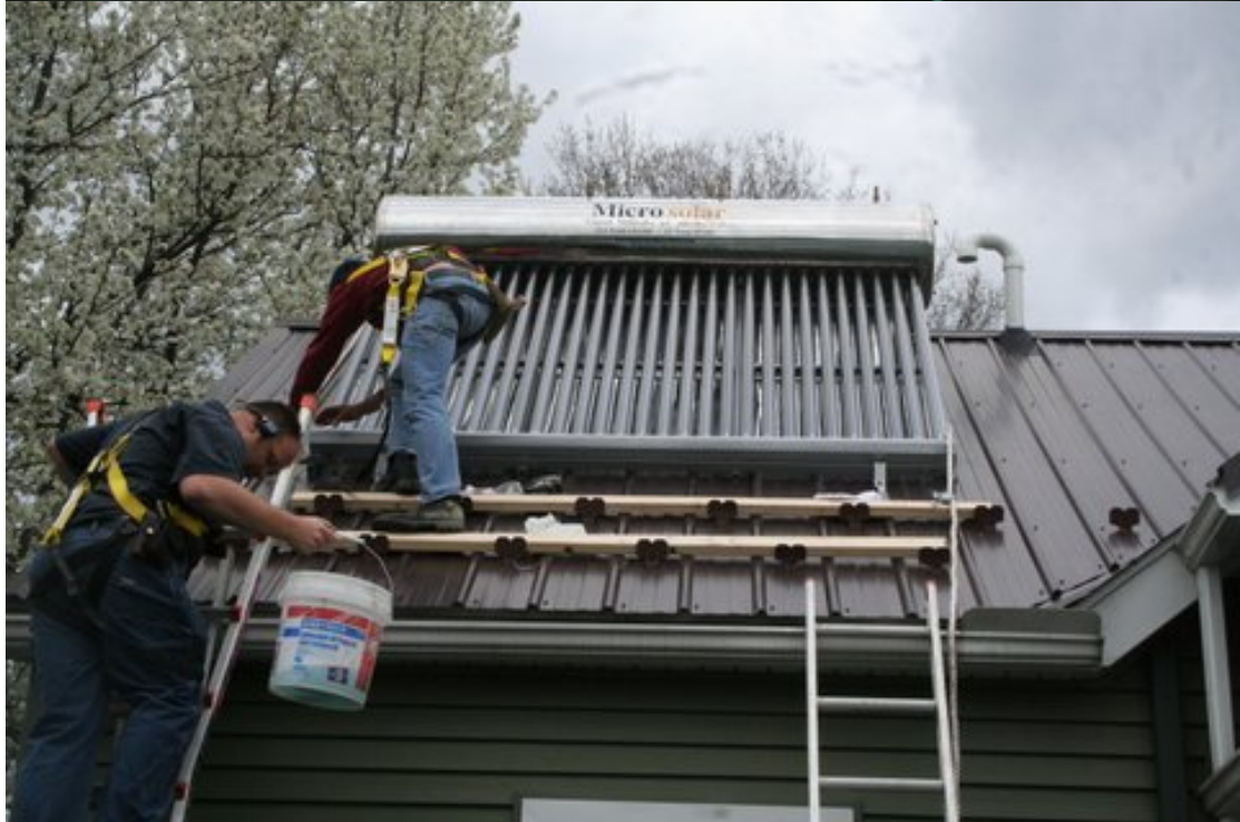
Potter House, Middleburg PA May 2014 Filling the Microsolar heater. By Affordable Fuels PA.
